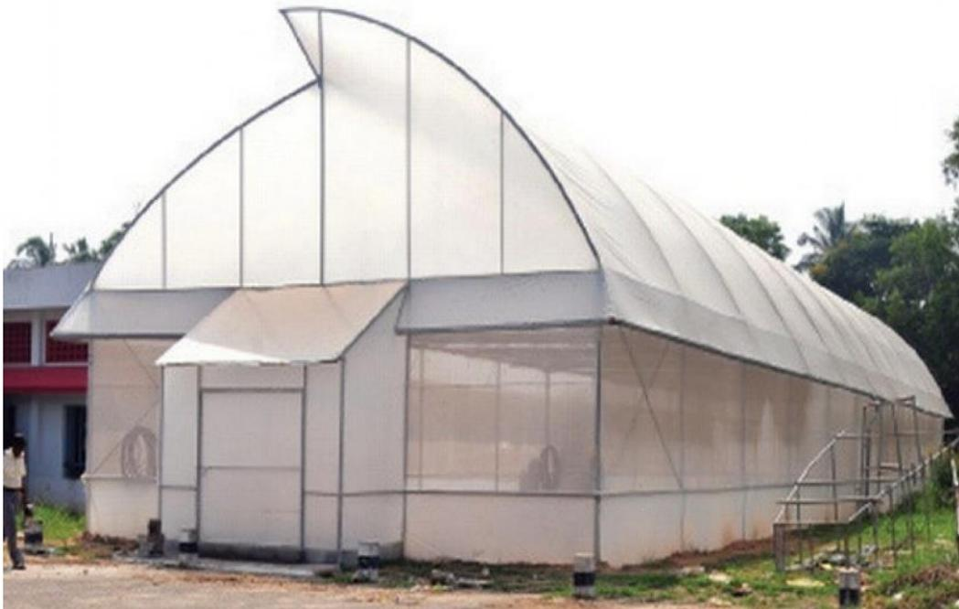
Polyhouse is a structure made of translucent material like polyethylene where the crops grow and develop under controlled climatic conditions. In developing countries like India polyhouse is a popular greenhouse technology due to its low cost of construction and easy maintenance. Polyhouse is cheaper as compared to greenhouse but the latter is more long lasting than polyhouse.
